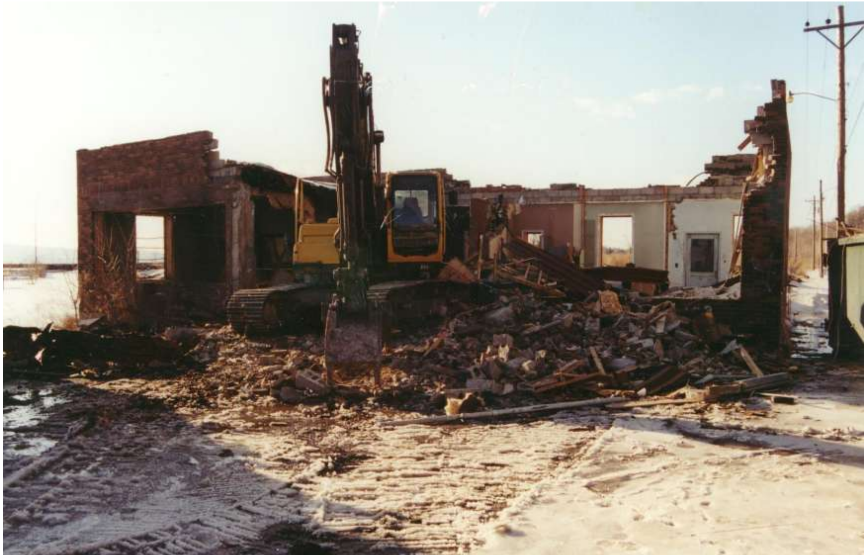
This building on the Urban Reserve was demolished in 1999 along with a small warehouse and loading platforms as part of the cleanup of a former fueling station
